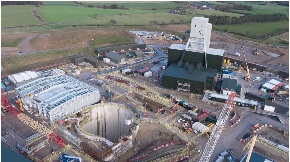
Figure 2.1 Woodsmith Project: Minehead site - progress with shaft sinking activities
